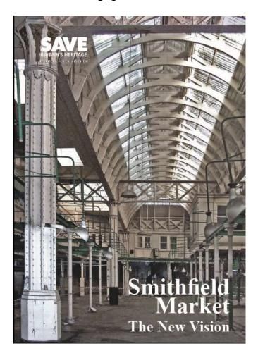
The existing interior consists of handsome parallel ranges of arched truss roofs with toplighting and louvred ventilation supported on X-trusses and tall 'Phoenix' columns.
