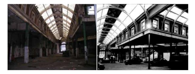
Like the General Market this has arched toplit roofs arranged as a triangular arcade reflecting the site. The Henderson view shows the major part of Horace Jones's trusses and arcades stripped out and an entirely new roof introduced, half of it aping the historic construction but clearly a modern fabrication supported on drainpipe columns.
